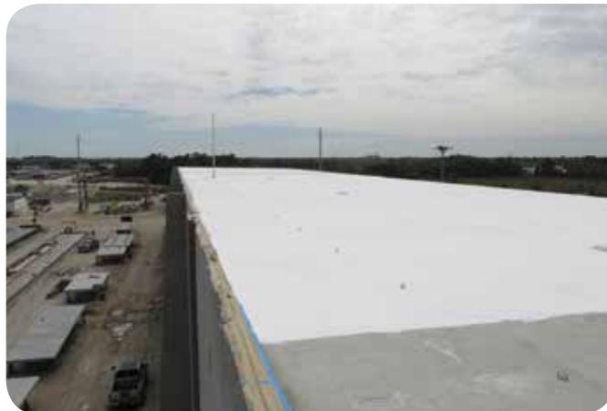
Over the course of three weeks, the crew members finished the system. They pressure-washed the roof and then spray-applied two passes of the WeatherBloc-IC to achieve an average dry film thickness of 20 mils (508 microns).
