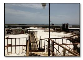
tanks well insulated but the harsh marine environment has not been able to attack the tanks and the tops are in the same condition as the day the coating was installed.
