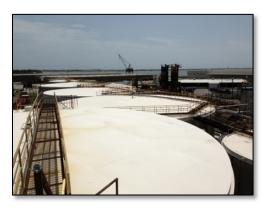
In Morehead City, NC, a bulk asphalt storage facility was looking to re-insulate many of their tank tops. They had noticed that over time the tops of the tanks had corroded and deteriorated to the point where something needed to be done to help protect them or they would run the risk of the tops needing complete replacement in just a few short years.
