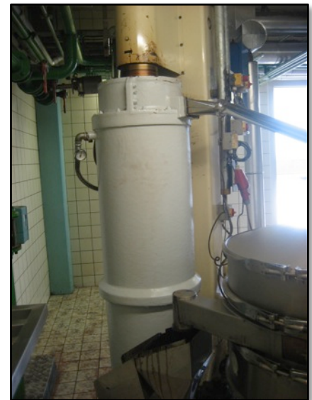
Crusher after being coated with non-flammable DTI
