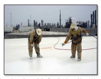
application, the coating's ability to withstand weather and the fact that it would provide an excellent radiant barrier, Calpine decided to apply the coating to the tank top.
