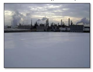
After the substrate was sandblasted and primed with Amerlock 400, 40 mils of Mascoat Industrial-DTI was applied in two successive coats by a crew of 4 men. A total of 5 days was needed to coat the entire roof of the tank.
