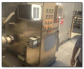
A geothermal plant in the desert was having trouble with the circuits in their electrical boxes. During the day, the sun was heating the stainless steel boxes to over 155°F (68.3°C), which was causing some of the internal circuits to overload. The cost of these unexpected shutdowns was two fold. No only did they have the cost of parts and labor to do the repairs, but they also had to shutdown the processes the boxes were controlling.
