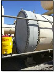
A geothermal plant in Southern California was having problems with the insulation on the end bells of their heat exchangers. They had to remove the end bells 2-4 times a year for maintenance on the internal tubes. Since they weighed approximately 9,000 pound, whenever they removed them and laid them on the ground, the insulation would be crushed. They, therefore, had to remove the insulation every time they remove the end bells. This was a very costly procedure.
