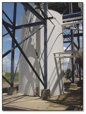
substrate. This effectively stops Corrosion Under Insulation, protecting the new heater, while at the same time providing the insulation abilities needed to keep the refinery process on schedule. It seemed to Mr. LeBlanc that this would solve all of his problems.
