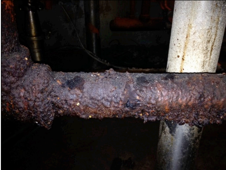
By-product of process baked on to pipes 6 months after application (above) and cleaned up after scraping (right). Notice contractor holding on with bare hand. Internal temperature approximately 250°F (121°C)
