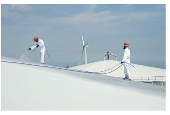
Before the Mascoat Industrial DTI application, the storage tank top was insulated with Poly Ureathane Foam (PUR). Because of the heavy atack of sea burds, CUI,(fire) Safety and qutility issue's BP decided to switch to the Mascoat solution.
