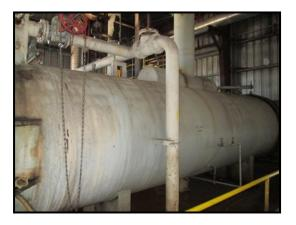
The evaporator on the right was coated with 80-100 mils (2.0-2.5 mm) of Mascoat Industrial-DTI, while 2.5-3 inches (63-76 mm) of mineral wool was installed on the one on the left. The facility did this to test the performance of the coating versus the mineral wool. When the plant is running, they operate between  $212^{\circ}-215^{\circ}F$  ( $100^{\circ}-102^{\circ}C$ ). During trial periods, no discernable difference in energy use was noted.
