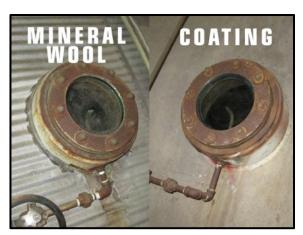
These reheaters were subject to a similar test like the evaporators above. The one on the left has 2.5" (63 mm) of mineral wool and the one on the right has approximately 120 mils (3 mm) of Mascoat Industrial-DTI. No discernable difference has been noted in the performance, but the plant manager said that they have to perform regular maintenance on the conventional insulation. They have had to do very little to the one with the insulating coating.
