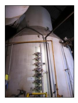
The vacuum pans are on the lower end of the temperature range found in this sugar mill. Operating at temperatures between 165–170°F (73–77°C), the sugar boils and results in crystallization. As you can see in the pictures above, these indoor pieces of equipment consist of very complex geometry that are very difficult to conventionally insulate. Along with the labor involved, there are many areas where moisture can intrude and promote CUI (flanges, inspection ports, support beams, etc.)
