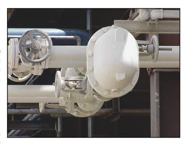
custom-tailored for each job. Since the valve assembly was very intricate, conventional insulation would need to be designed before being fabricated, increasing costs and time. Conventional insulation would also do little to protect the expensive valve from CUI.
